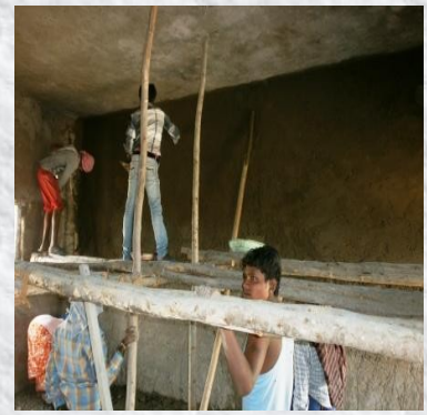
workmen doing the plastering of the walls in the high school
